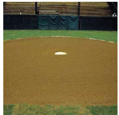
STEP 6: Level and compact the new surface. Add Diamond Pro® Infield Conditioner to the finished area for a professional quality playing surface.
