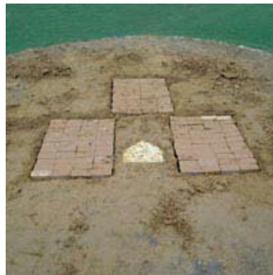
STEP 5: Fill in the 1/2" remaining area with either the cut out loose material or with Diamond Pro® Mound / Home Plate Clay for the ideal surface.
