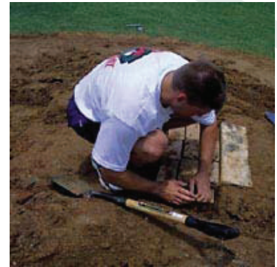
STEP 3: Place Diamond Pro® Mound / Home Plate Clay Bricks as evenly and close together as possible.
